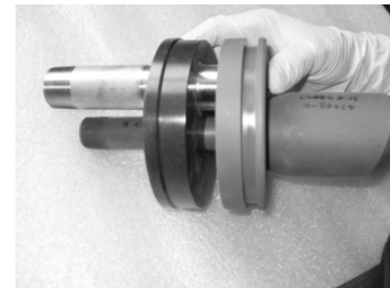
Installing the Bearing Plate and Sealing Plate
